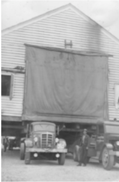
It took 2 trucks to move the chapel.
